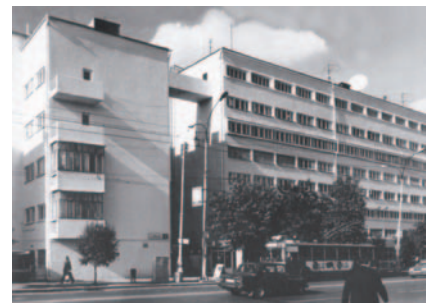
3/ Jan Brinkman, Leendert van der Vlugt: Van Nelle factories, Rotterdam 1925–1931 4/ Moisei Ginzburg, Alexander Pasternak: housing complex, 1929–1931 Ekaterinburg photo selection from the Docomomo registers
