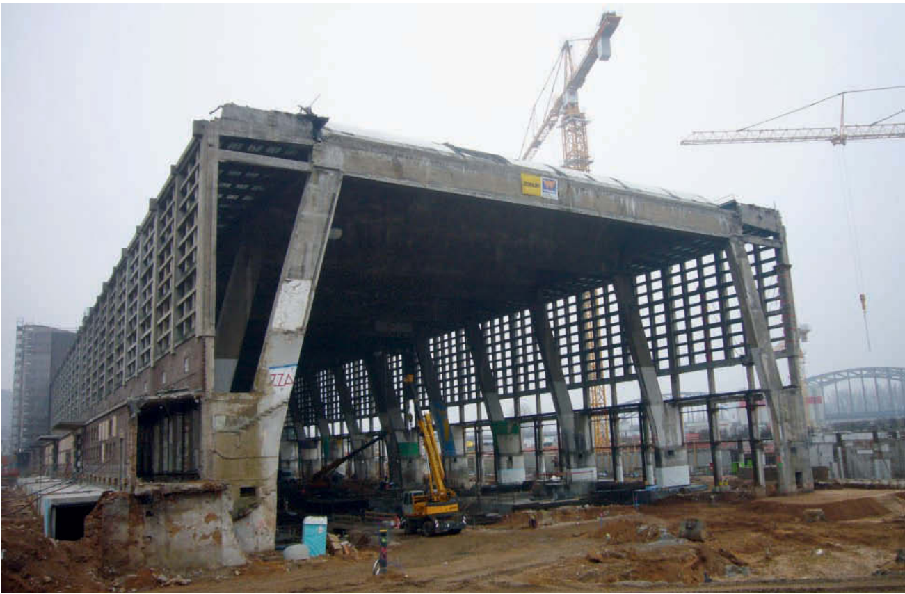
Building site at the former wholesale fruit and vegetable market by M. Elsaesser, 1926–28, for the ECB headquarters by Coop Himmelb(l)au, Frankfurt // photo Monika Platzer
