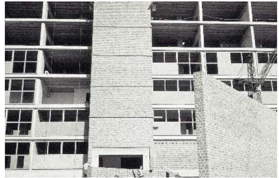
Installation of the prefabricated elements // photo Willy Van Der Meeren Archives
