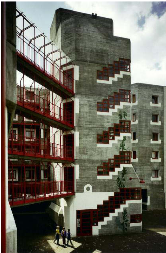
Staircase tower to balcony access apartments // photo Inge and Arved von der Ropp, Kirchanschöring
