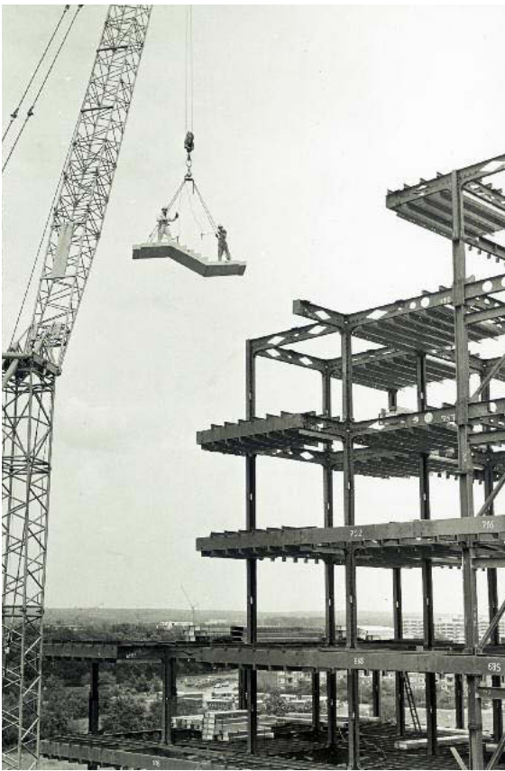
Construction photo // Richard J. Dietrich Archives, Traunstein
