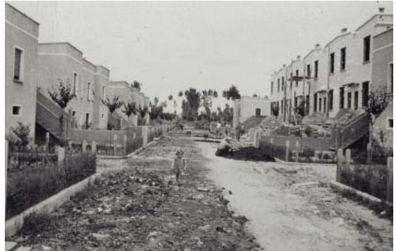
View of the green areas between the houses
