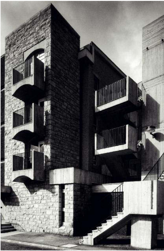
View of external stairs leading to 2 Brown's Close // photo Henk Snoek, 1969
